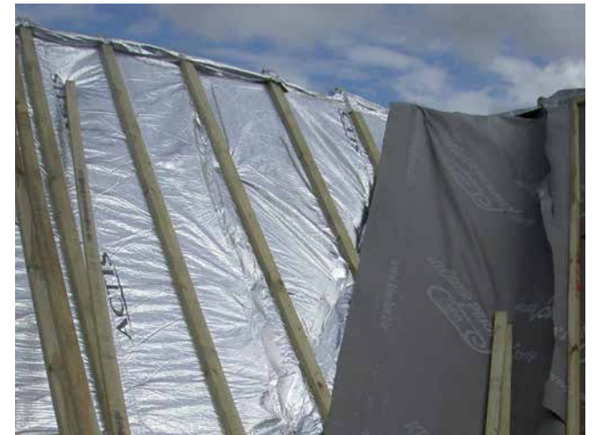
Images Bottom and Top Right: Enhanced insulation to roofs can be achieved by re-slatting using modern multi-foil insulation materials.
